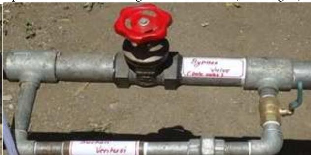
**Fig. 8:** Bypass valve in parallel with suction venturi
